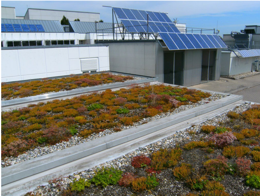
Extensives GD: 9 cm, Sedum, 2011
